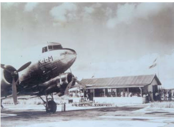
PJIA's first terminal building in 1943
