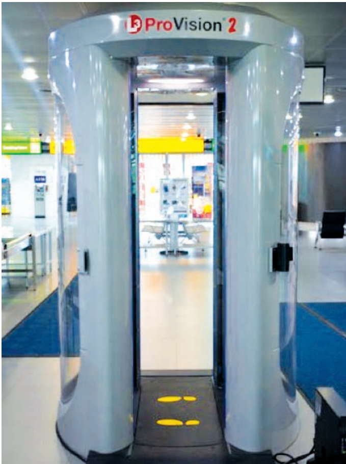
L-3 ProVision security screening machine installed at SXM Airport.
