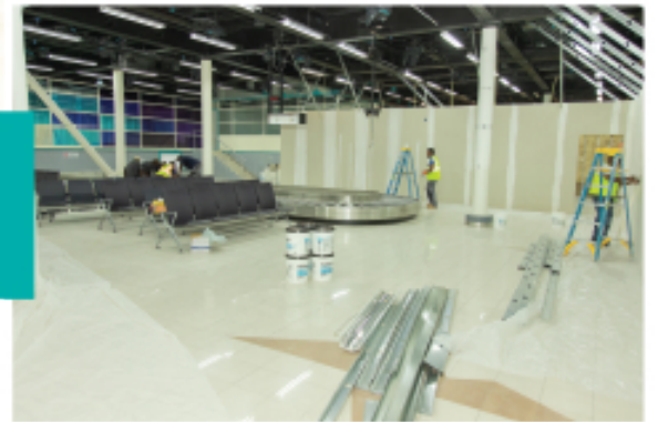
Image 2: Ongoing works at the Package 1 - Temporary Operations terminal building.
