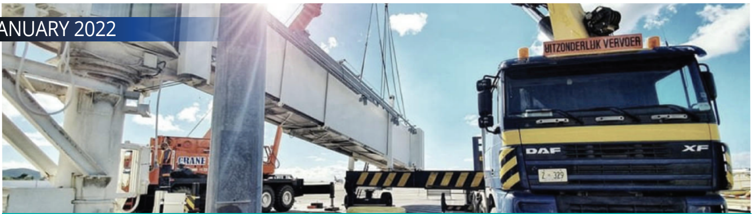
File photo of the removal of the Passenger Board Bridges at PJIA in 2020.
